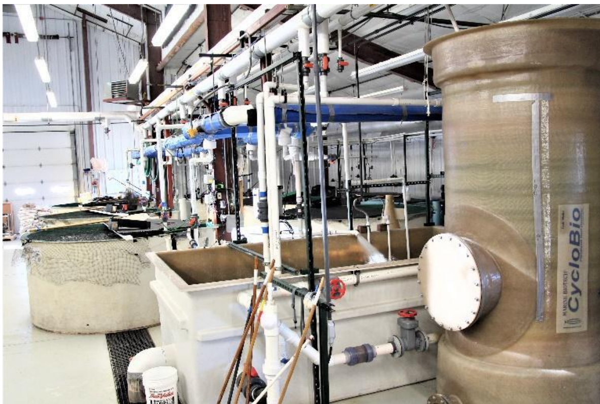
Figure 8. An Indoor Recirculating Aquaculture System
